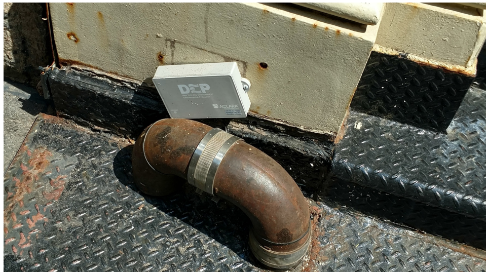
STOREFRONT EXPOSED EQUIPMENT
