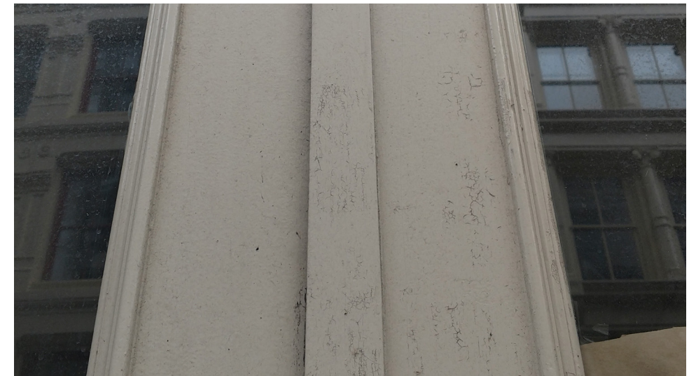
STOREFRONT DOOR WOOD FINISH CONDITION
