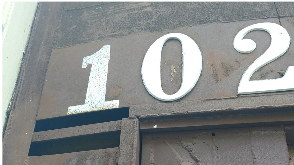
BUILDING ADDRESS CONDITION
