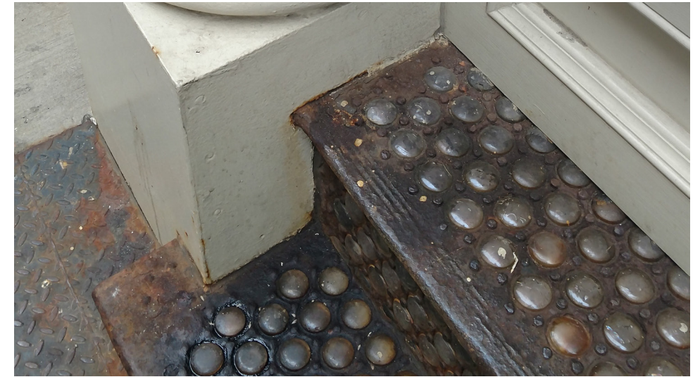
EXISTING PRISMATIC VAULT LIGHTS
